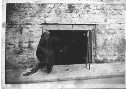
The entrance to "The Hole" before renovation
