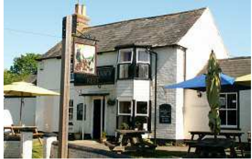
The Sportsman's Rest, Porchfield An Asset of Community Value
