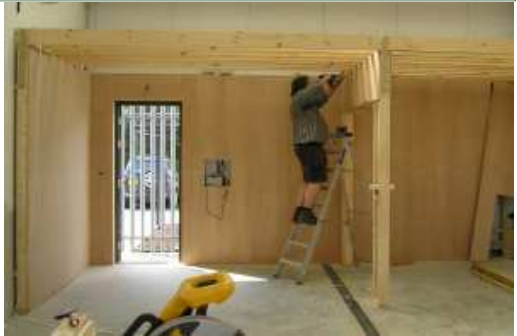
Jed Jackson busily preparing the new site
