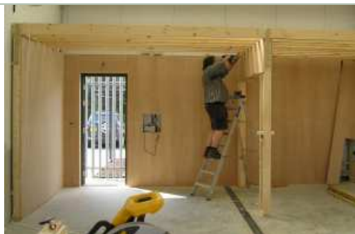
Jed Jackson busily preparing the new site
