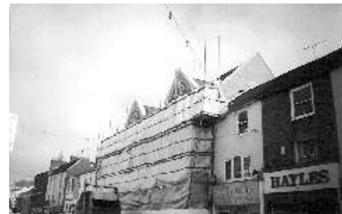
5. Which shop- front is under construction here?
