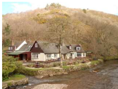
Fingle Bridge Inn
